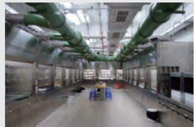
Color checking room
